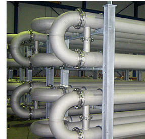
Mud heat exchanger 1.4571, double tube condition for heat recovery in a waste water treatment plant
